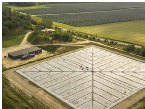
FIGUR 20: DAMVARMELAGER FOR SOLVARME I DRONNINGLUND (62.000 M3)
